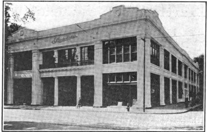
In this building in Detroit, Mich., the Studebaker Corporation has organized a model garage, salesroom and repair shop which is used for the purpose of educating its dealers and representatives all over the country
